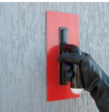
Application and finishing of Graffiato Silox by plastic trowel.
