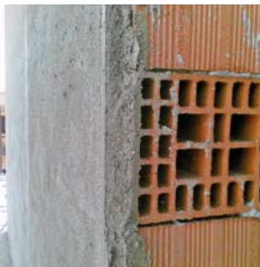
Example of application of Thermoisol plaster.
