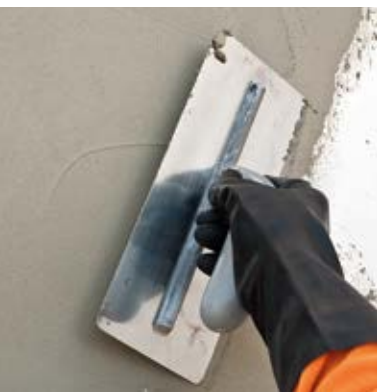
Application of Rasocem Pasta by smooth inox trowel.
