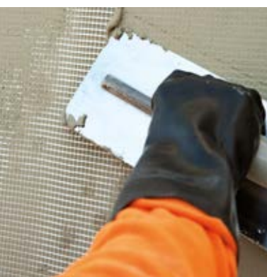
Burying of fibre glass mesh and second coat application of Rasocem Pasta.
