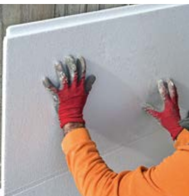
Application of thermal insulating panel
