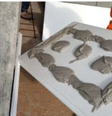
Application of Rasocem KR EXTRA on the reverse side of the panel
